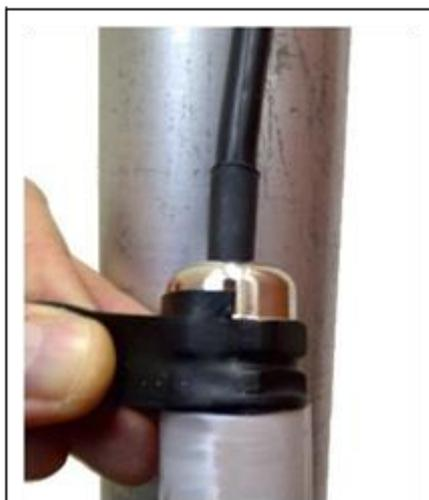
**Figure 104: Applying sealant tape to an external connection**
